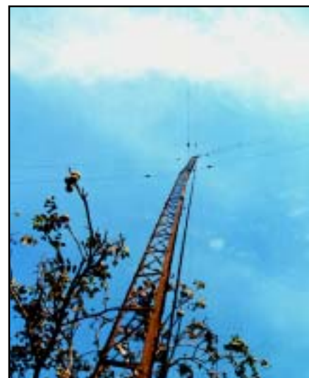
One of the towers, which have stood at the site in Warren County, Ohio, since 1950.
